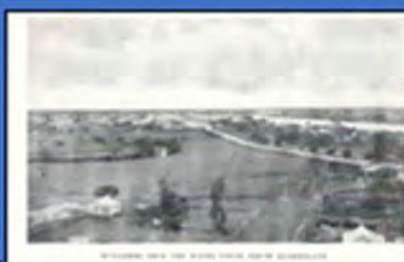
7. → BUNDABERG FROM THE WATER TOWER, SOUTH QUEENSLAND
