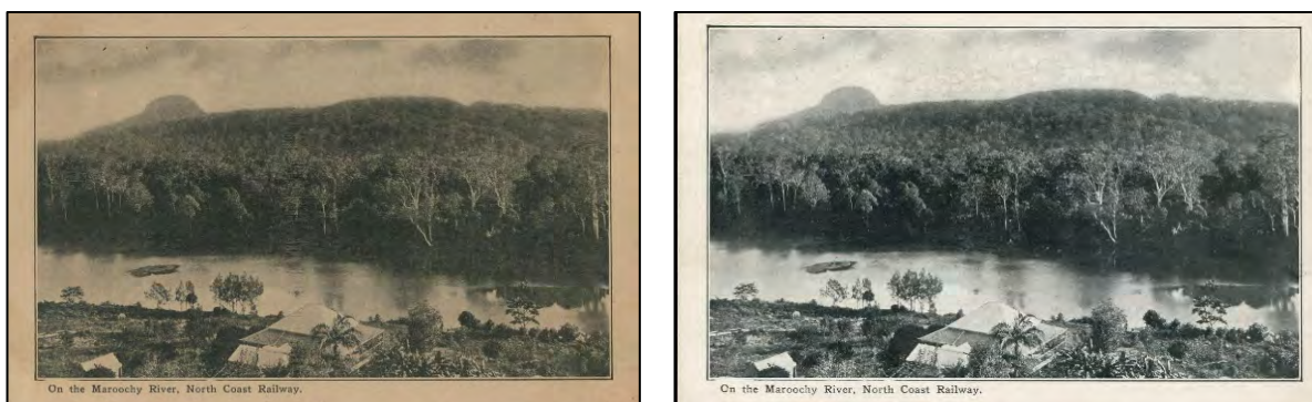
Figure 23 Proof on buff paper of On the Maroochy River, North Coast Railway Card (endorsed on reverse PROOF Ref. No. G1579/10) (left) and Figure 24 Issued Card (right)
