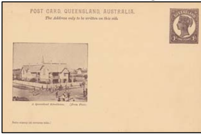
a. A Queensland Schoolhouse.
